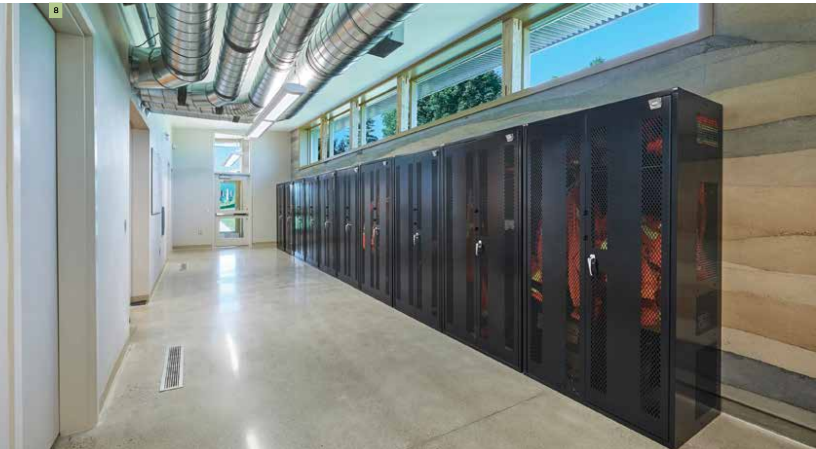
8. The clearstorey provides light and privacy in the locker room. In some areas the polished concrete floor contains broken glass and even some of the architect’s personal fossil collection.
